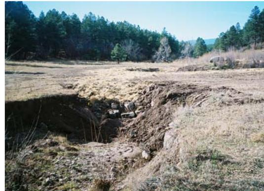
At the upper end of this work area were two more major head cuts one on each side of a earth tank berm. Several options were looked at and the one chosen was to rebuild the dam with an adequate spillway to accommodate a 25 year storm event.
