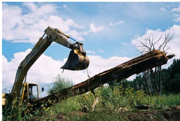
Mechanical work entailed 118 hours and 38 various structures were installed over three property owners. These included: Pat Jones, Stanly Lucero, and Elaine Speilman. Materials were found locally—boulders from a fire line created during a fire in 02', a hillside of glacial piled rock and trees toppled by wind, erosion and beaver. 4 point bars were also shaved to allow the stream more room to spill onto the flood plain and take pressure off the eroding outside stream banks.
