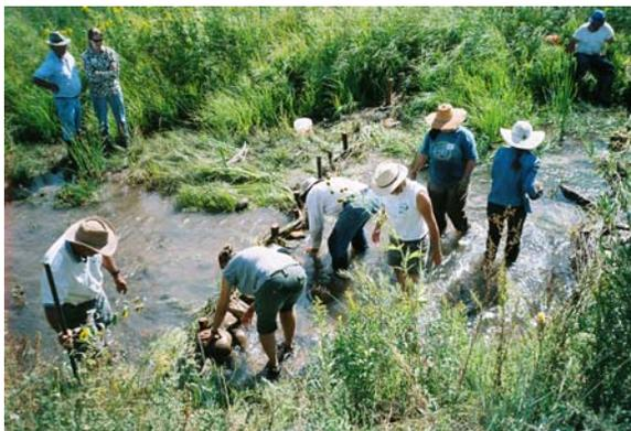
September, 05 induced meandering and stream bank stabilization work was completed on **3800'** of Manuelitas Creek. Most was done with heavy equipment, but a part was also completed with hand labor during an educational workshop held on the property. Picture to left, a cottonwood log vane being installed at Jones' property
