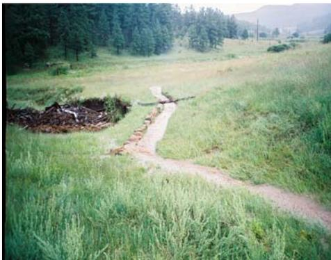
This last structure was built where we wanted to divert water again, from another arroyo (the logging road) on to flat land to help disperse the water more evenly. If we can break the single thread flow into numerous flows around the 40' edge of the lower outside rim of the half moon, the possibility of erosion is reduced completely.
