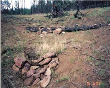
13 small rock check dams, some incorporating soil filled burlap bags along with one rock dams were installed to slow surface water flow, retain sediment and increase water infiltration. 4 log check dams and 3 larger boulder and rock check dams were constructed to reduce and heal erosion-taking place in several arroyos.
